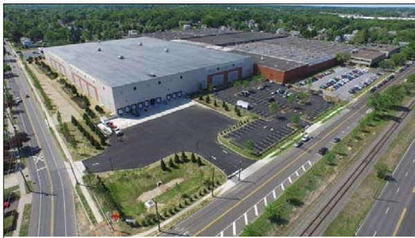
Simon & Schuster's newly expanded distribution center in Delran, NJ.
